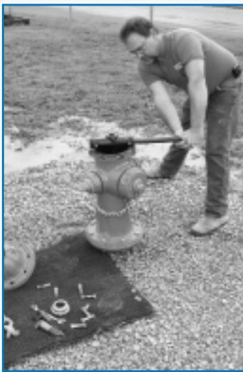
6. Use the manufacturer's seat wrench to unscrew the seat ring.
